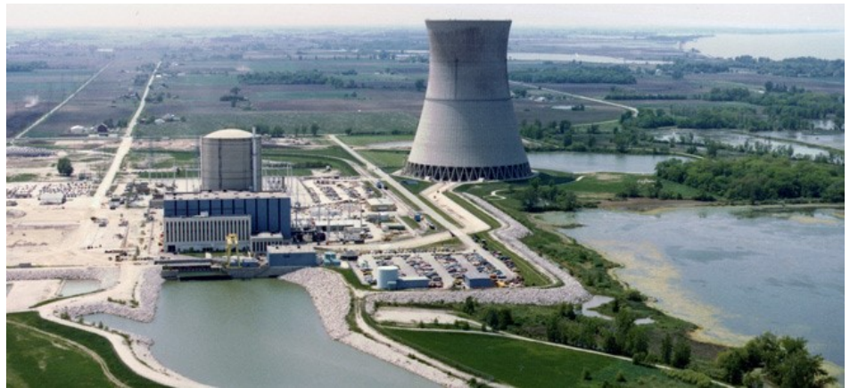
FirstEnergy's Davis-Besse nuclear plant
