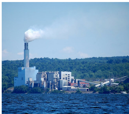
Cayuga power plant
